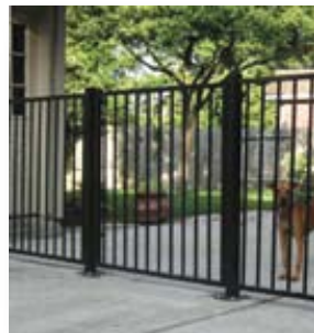
2 RAIL FENCE STYLE WITH SINGLE SWING GATE
